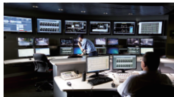
Command and control center
