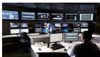
Command and control center
